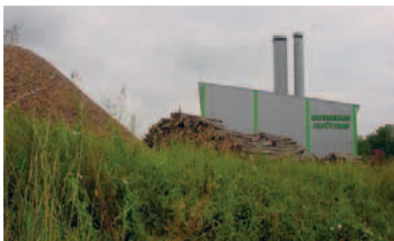
Photo: Biomass district heating station (City of Altötting)
